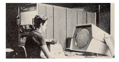
*User at the console of the Digital Equipment Co. PDP-1 computer. (Source: Digital Equipment Corp.)*
