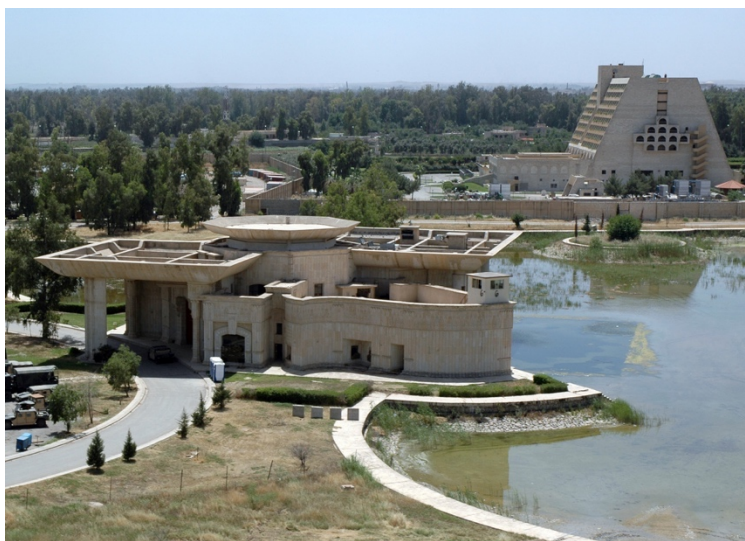
Image of Saddam's Palace in Ninawa, one of the palaces used by Saddam Hussein in Mosul, northern Iraq, Ninawa (Nineveh) province. US Army Corps of Engineers (USACE) photograph by ACoE photographer Jim Gordon, C.C.O, via Wikimedia Commons.
