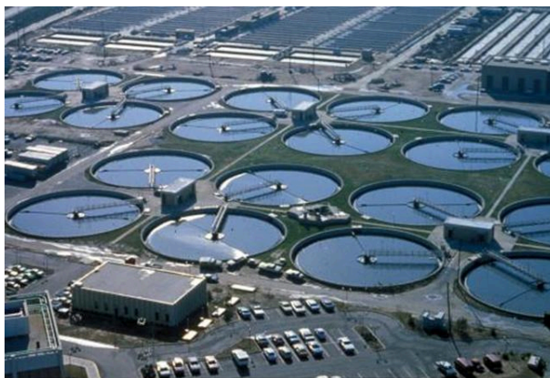
Figure 6.4.6. Wastewater treatment facilities, such as this one, remove contaminants from wastewater before the water is released back into the natural environment. (credit: “eutrophication&hypoxia”/Wikimedia Commons)
