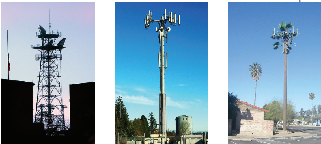
Figure 8.1.3. Radio and cell towers are typically used to transmit long-wavelength electromagnetic radiation. Increasingly, cell towers are designed to blend in with the landscape, as with the Tucson, Arizona, cell tower (right) disguised as a palm tree. (credit left: modification of work by Sir Mildred Pierce; credit middle: modification of work by M.O. Stevens)
