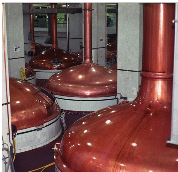
Figure 1.2.8. An oxide of carbon is removed from these fermentation tanks through the large copper pipes at the top. (credit: “Dual Freq”/Wikimedia Commons)
