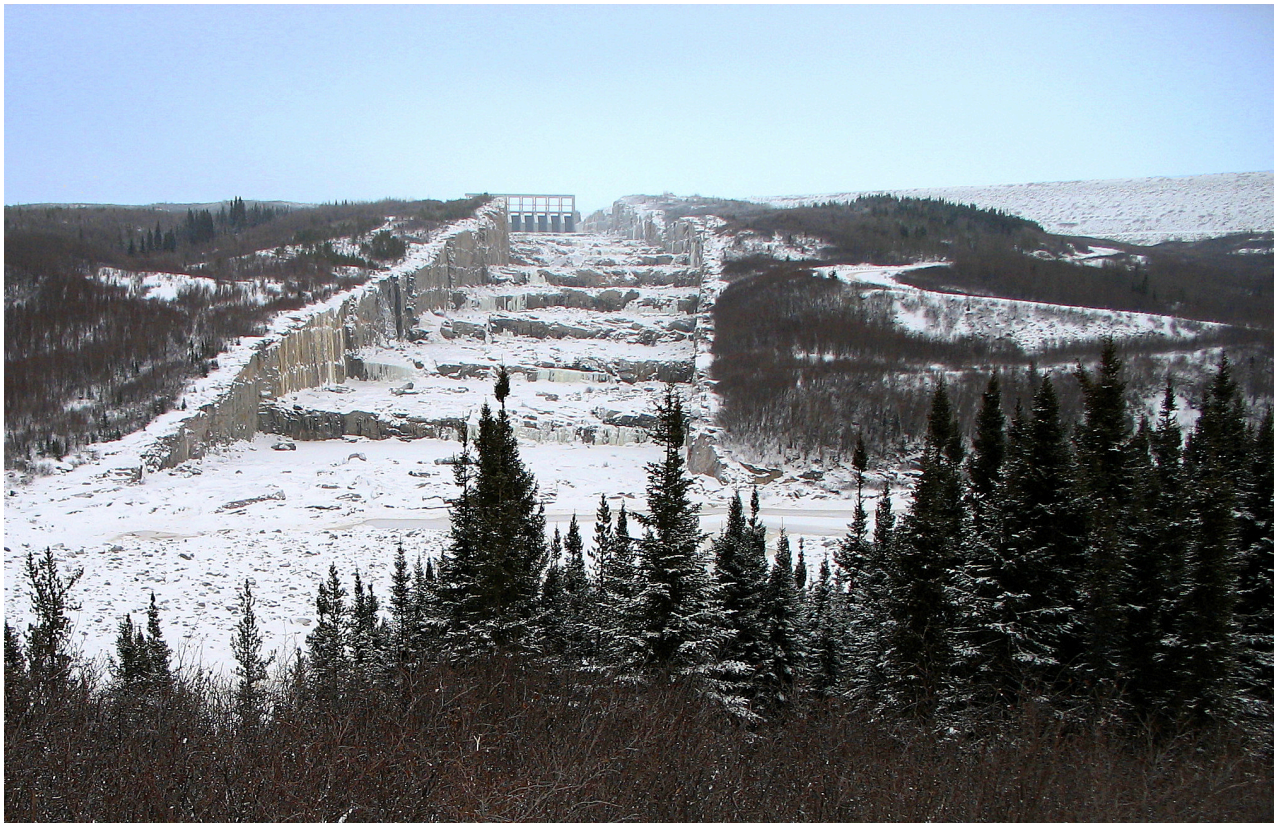
The spillway of the Robert-Bourassa Dam (formerly La Grande-2). This dam was one of the dams in the James Bay Projects. Photo by: P199 at Wikimedia Commons. (CC BY 2.5) & (CC BY-SA 3.0) [104]
