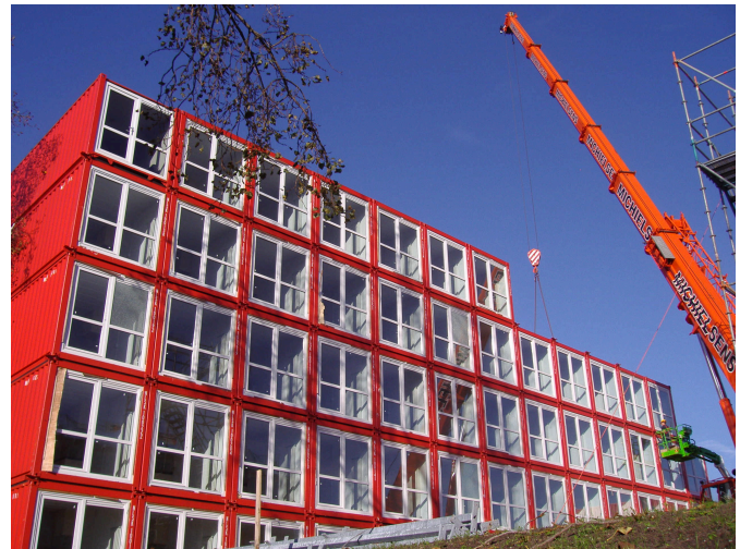
Project Keetwonen Amsterdam creates 1000 student apartments built out of shipping containers. Photo credits to: Tempohousing. Text and image reproduced with permission from Tempohousing [137]
