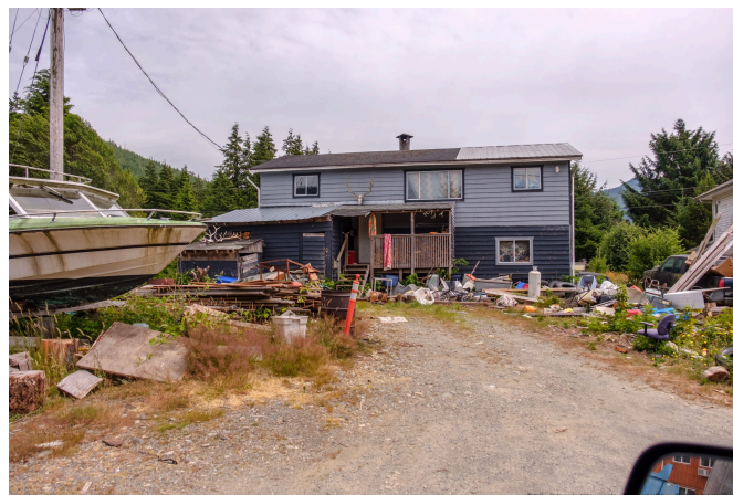
House in need of serious repair, Malachan Indian Reserve, Vancouver Island (2017) Credits to: Mikofox Photography (CC BY-NC-SA 2.0) [135]
