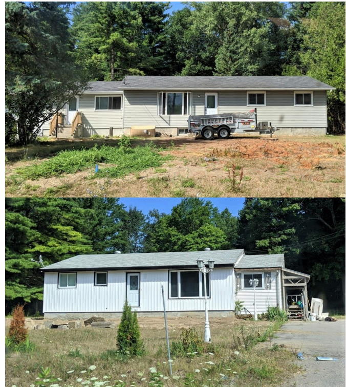
Typical on-reserve housing units. 3 bedroom and 2 bedroom bungalows located on Tyendinaga Mohawk Territory, Ontario. Photo credits to: Pauline Galoustian (Public Domain) [134]
