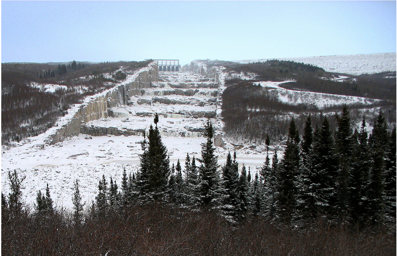
The spillway of the Robert-Bourassa Dam (formerly La Grande-2). This dam was one of the dams in the James Bay Projects. Photo by: P199 at Wikimedia Commons. (CC BY 2.5) & (CC BY-SA 3.0) [104]
