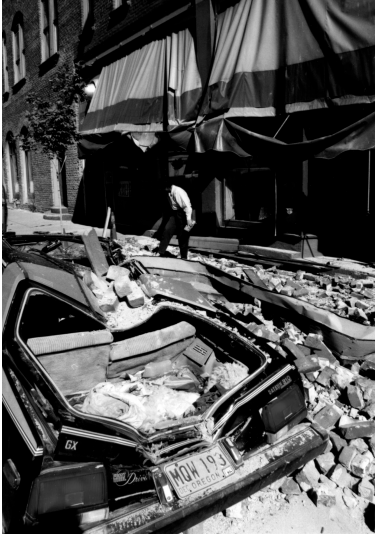
Figure 6-25. Downtown Klamath Falls, Oregon, after the earthquakes of September 20, 1993. Automobile parked in front of Swan's Bakery was crushed by falling bricks from an unreinforced parapet.
