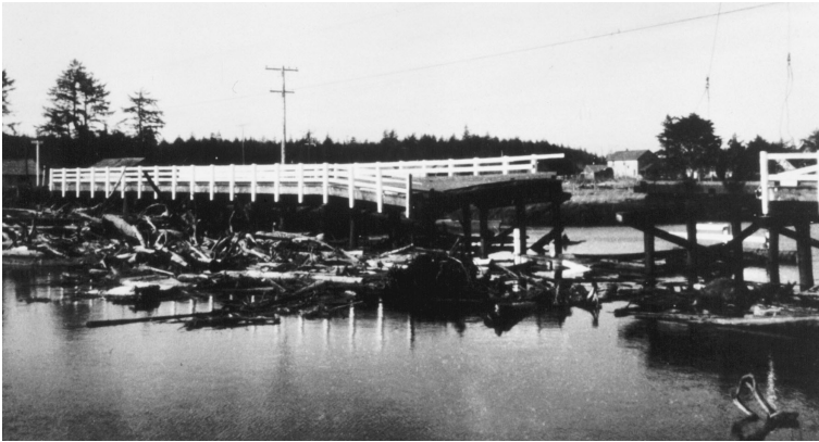
Figure 9-2. Bridge across Copalis River, Washington, destroyed during the tsunami accompanying the 1964 Good Friday Earthquake in southern Alaska.
