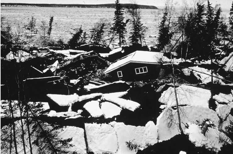
Figure 8-7. Destruction of part of Turnagain Heights subdivision of the city of Anchorage by liquefaction of a sand layer in the Bootlegger Clay accompanying the Good Friday 1964 Earthquake in the Gulf of Alaska. The ground and the houses were disrupted; note the tilted trees. Photo by George Plafker, USGS
