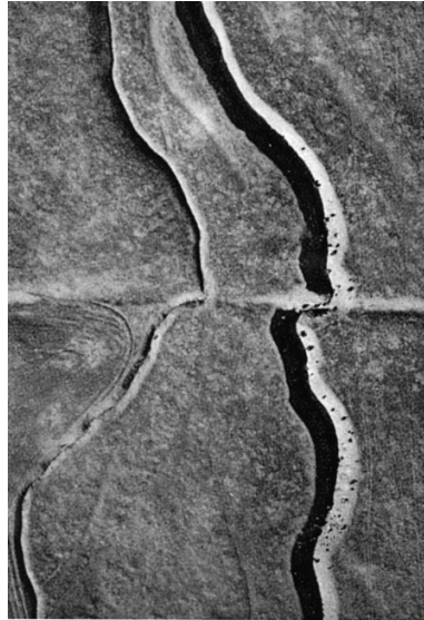
Figure 3-5b. Right-lateral strike-slip fault. Offset furrows in a cultivated field near El Centro, California, during an earthquake on October 15, 1979.
