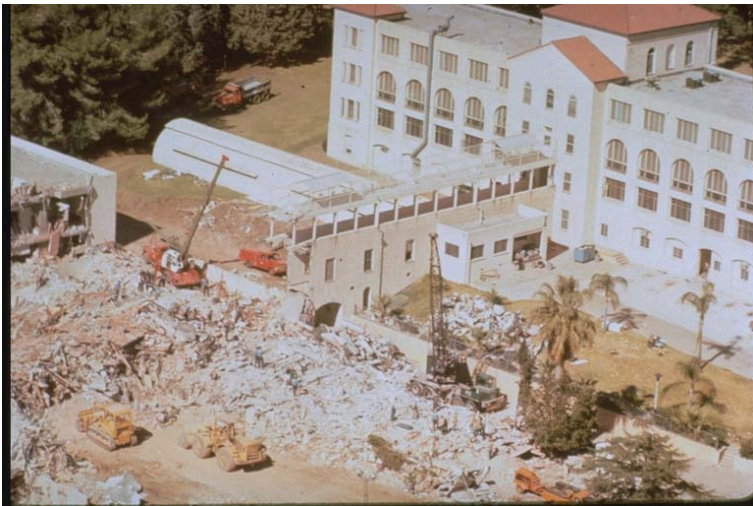
Figure 12-1. Aerial view of the damage to the San Fernando Veterans Administration Hospital campus after the 1971 Sylmar, California Earthquake. Forty-seven of the sixty-four deaths attributed to the earthquake were a result of the collapse of this structure, built in 1926, before earthquake-resistance building codes were adopted. Adjacent building, constructed after building codes were upgraded after the 1933 Long Beach Earthquake, did not collapse. Photo by E. V. Leyendecker, U.S. Geological Survey
