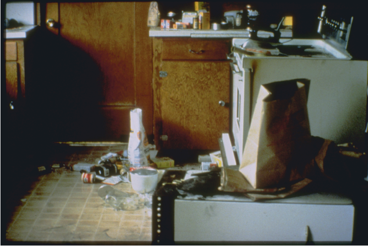
Figure 11-9. Damage to contents of the kitchen in a residence in Petrolia, California, as a result of the 1992 Cape Mendocino Earthquake. Appliances shifted several inches away from the wall. All items were shaken off the shelves with considerable glassware breakage. Photo courtesy of National Oceanic and Atmospheric Administration.
