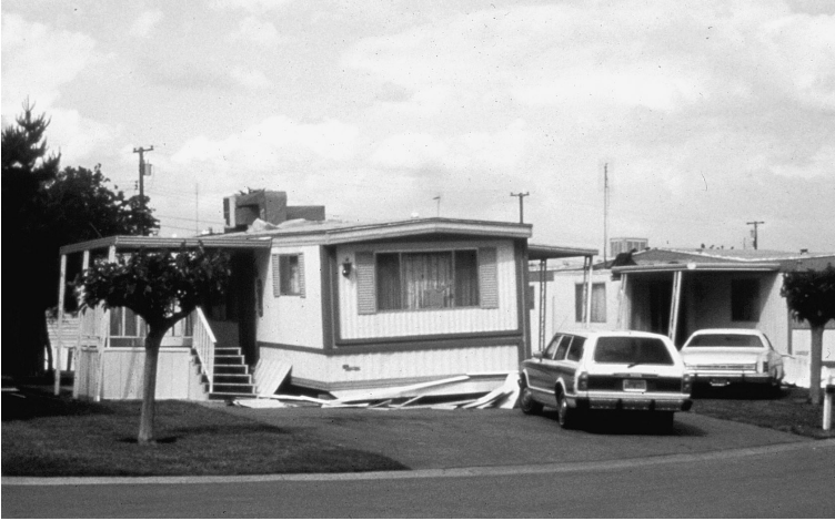
Figure 11-18. Mobile home has slid off its supports during an earthquake. Photo courtesy of California Office of Emergency Services
