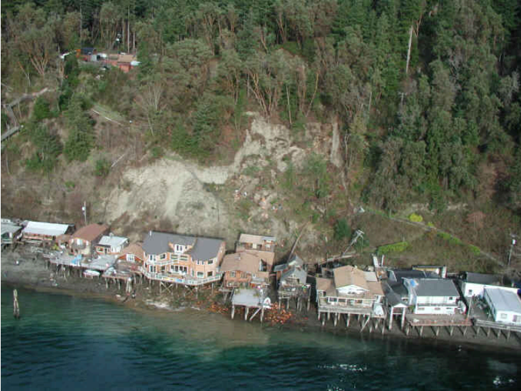
Figure 8-12b. Salmon Beach landslide near Tacoma Narrows after the 2001 Nisqually earthquake. Houses overlooking Puget Sound have no road access; landslide struck behind the houses, as it did in 1949. Photo courtesy of Jon Bray, University of California Berkeley.
