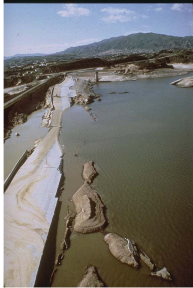
Figure 12-16. Van Norman Dam, San Fernando Valley, California, after the 1971 Sylmar Earthquake. About eight hundred thousand yards of the embankment, including the parapet wall, dam crest, most of the upstream slope, and a portion of the downstream slope, slid into the reservoir, causing a loss of about thirty feet of dam height. Fortunately, the dam was only about half full at the time. Eighty thousand people living downstream from the dam were ordered to evacuate, and steps were taken to lower the water level in the reservoir. Photo by E. V. Leyendecker, USGS
