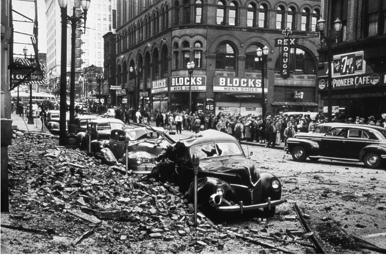
Figure 5-5. Yesler Way, downtown Seattle, showing damage in 1949 earthquake from falling parapets and brick ornamentation and a collapsed fire escape, shown at left. Photo by George Cankonen, Seattle Times
