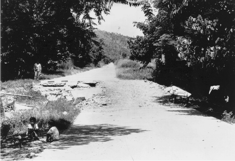
Figure 3-6. Road displaced to the left during an earthquake in 1990 on a left-lateral strike-slip fault on the Island of Luzon in the Philippines.
