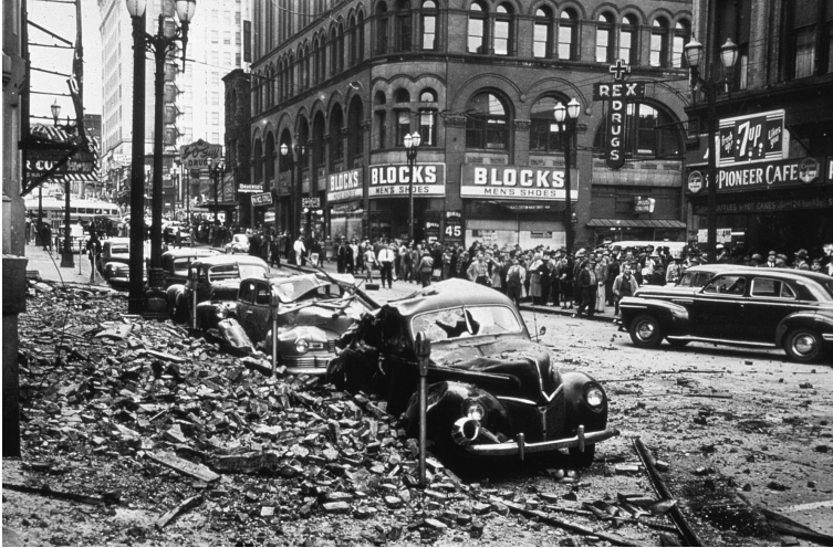
Figure 5-5. Yesler Way, downtown Seattle, showing damage in 1949 earthquake from falling parapets and brick ornamentation and a collapsed fire escape, shown at left. Photo by George Cankonen, Seattle Times
