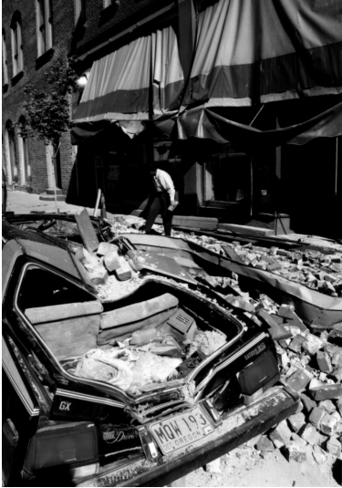
Figure 6-25. Downtown Klamath Falls, Oregon, after the earthquakes of September 20, 1993. Automobile parked in front of Swan's Bakery was crushed by falling bricks from an unreinforced parapet.
