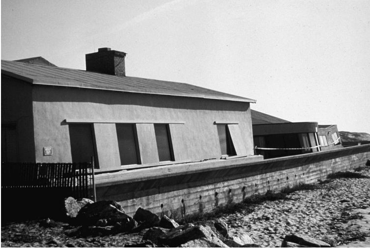
Figure 8-6. Tilted buildings at San Jose State University Marine Laboratory at Moss Landing, California, due to liquefaction of beach deposits during the October 1989 Loma Prieta Earthquake. Photo by G. W. Wilson, USGS
