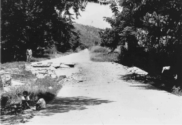
Figure 3-6. Road displaced to the left during an earthquake in 1990 on a left-lateral strike-slip fault on the Island of Luzon in the Philippines.
