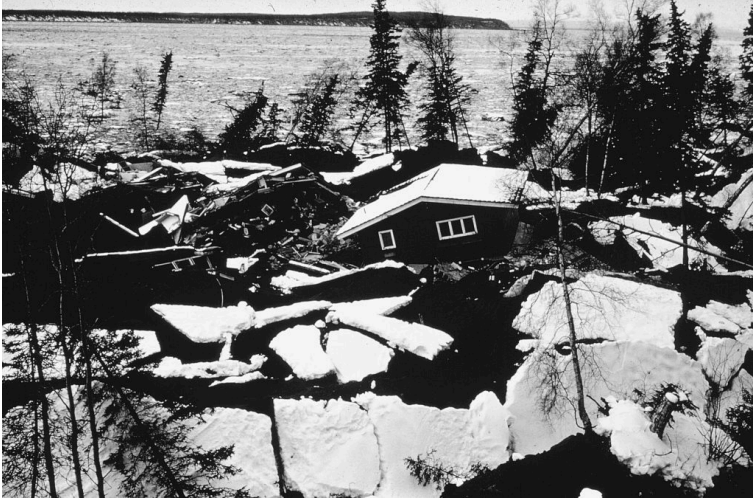
Figure 8-7. Destruction of part of Turnagain Heights subdivision of the city of Anchorage by liquefaction of a sand layer in the Bootlegger Clay accompanying the Good Friday 1964 Earthquake in the Gulf of Alaska. The ground and the houses were disrupted; note the tilted trees. Photo by George Plafker, USGS
