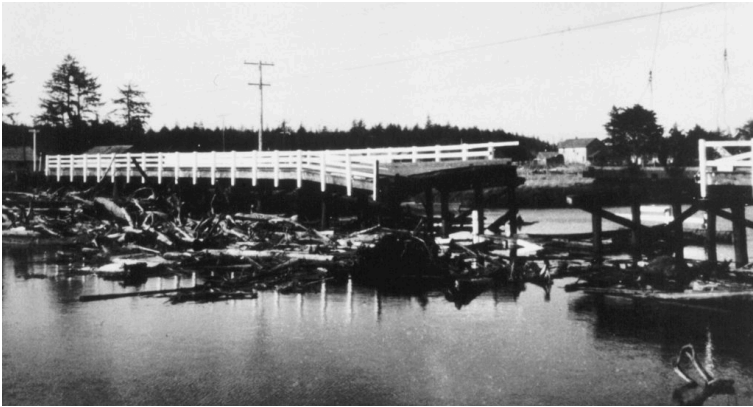
Figure 9-2. Bridge across Copalis River, Washington, destroyed during the tsunami accompanying the 1964 Good Friday Earthquake in southern Alaska.
