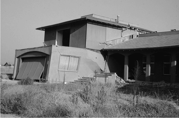
Figure 11-16. Split-level house in Crestview Tract, San Fernando Valley, showing failure of the connection between the single story (right) and the two-car garage with bedrooms above. Note the difference in height between the front steps and the single story, indicating cripple-wall failure of the single story. Photo by Robert Yeats
