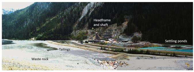
Figure 20.1.10 The tailings pond at the Myra Falls Mine on Vancouver Island. The dry rock in the middle of the image is waste rock. Myra Creek flows between the tailings pond and the headframe. The settling ponds (right) are used for processing water from the concentrator.
