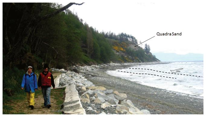
Figure 17.3.4 The Quadra Sand cliff at Comox, and the extensive concrete and rip-rap barrier that has been constructed to reduce erosion. Note that the waves (dashed lines) are approaching the shore at an angle, contributing to the longshore drift.
