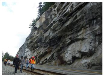
Figure 15.2.4 Site of the 2008 rock slide at Porteau Cove. Notice the prominent fracture set parallel to the surface of the slope. The slope has been stabilized with rock bolts (visible near to the top of the photo) and holes have been drilled into the rock to improve drainage (one is visible in the lower right). Risk to passing vehicles from rock fall has been reduced by hanging mesh curtains (background).
