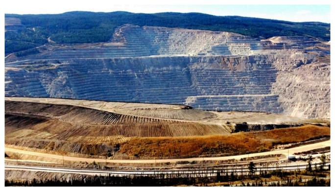
Figure 20.0.1 The open pit (background) and waste-rock piles (middle) of the Highland Valley Copper Mine at Logan Lake, British Columbia.
