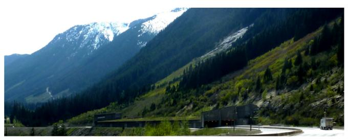
Figure 15.3.5 A snow avalanche shelter on the Coquihalla Highway. The expected path of the avalanche is the steep un-treed slope above.
