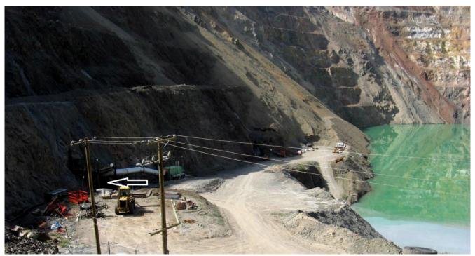
Figure 20.1.9 Entrance to an exploratory decline (white arrow) for the New Afton Mine situated in the side of the open pit of the old Afton Mine, near Kamloops, B.C.
