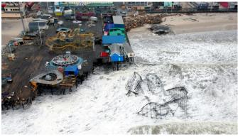
Figure 19.3.2 Damage to the Casino Pier, Seaside Heights, New Jersey, from Hurricane Sandy, November 2012.
