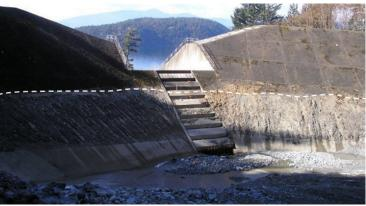
Figure 15.3.6 Two strategies for mitigating debris flows on the Sea-to-Sky Highway. Left: A concrete —lined channel on Alberta Creek allows debris to flow quickly through to the ocean. Right: A debris-flow catchment basin on Charles Creek. In 2010, a debris flow filled the basin to the level of the dotted white line.
