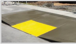
A sidewalk ramp
