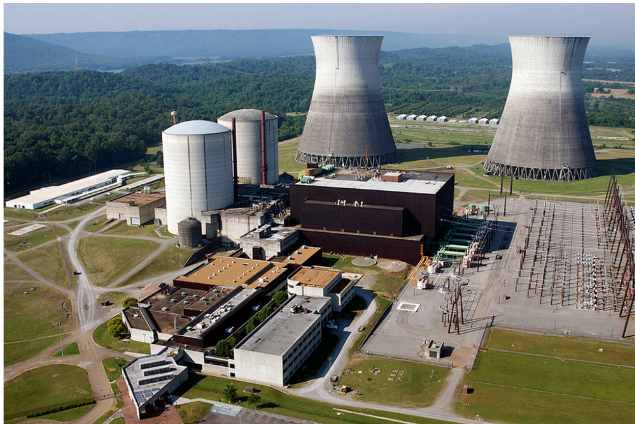
Figure 10.17 The Phillipsburg Nuclear Power Plant in Germany uses a fission reactor to generate electricity.
