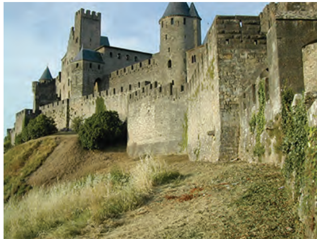
Figure 1.13 One of the most beautifully preserved medieval walled cities is Carcassonne, France. Notice the use of a double wall.
