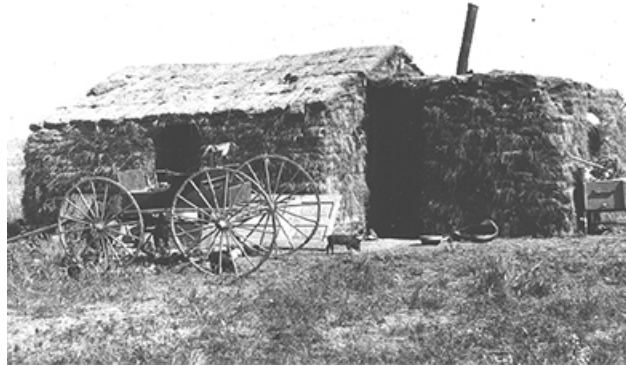
Figure 17.8 Sod houses were common in the Midwest as settlers moved west. There was no lumber to gather and no stones with which to build. These mud homes were vulnerable to weather and vermin, making life incredibly hard for the newly arrived homesteaders.
