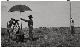
A leveling crew at work in 1916. (Hodgson, 1916).
