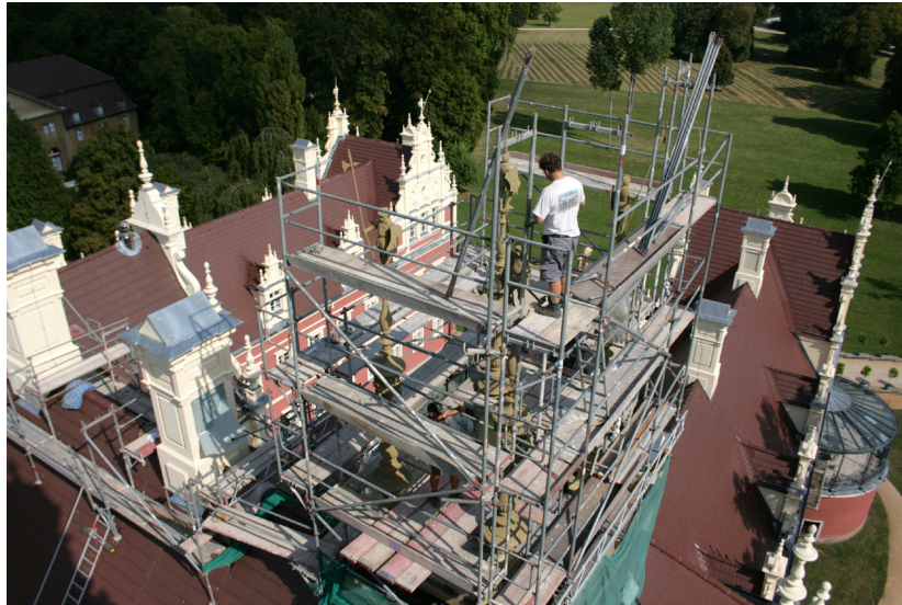
Figure 5 — A typical tube and clamp scaffold
