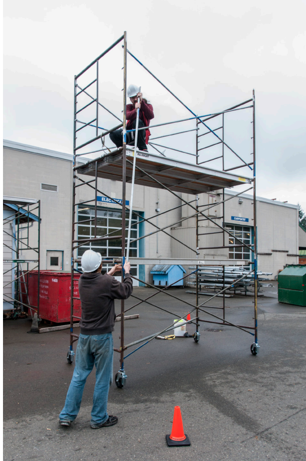
Figure 20 — Erecting a welded steel scaffold frame
