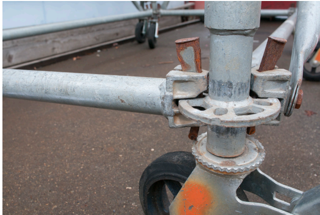
Figure 2 — Ledger and standard connection
