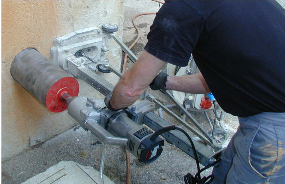
Figure 24 — Core drilling
