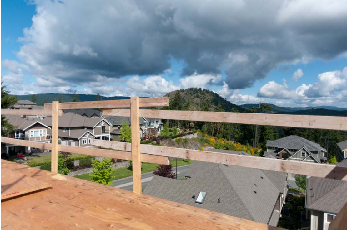
Figure 5 — Guardrail and midrail
