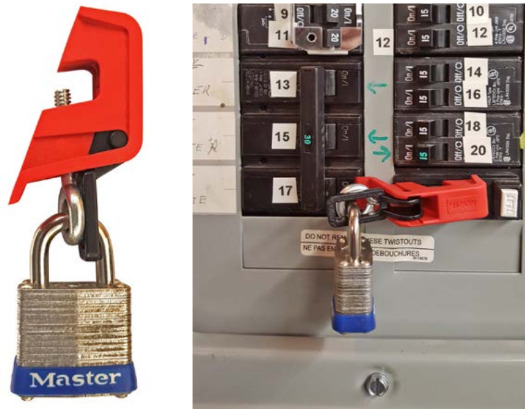
Figure 5 — Breaker lockouts
