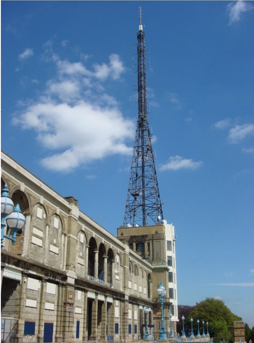
Figure 6.2.3 BBC television studio and radio transmitter, Alexandra Palace, London Image: © Copyright Oxyman and licensed for reuse under a Creative Commons Licence
