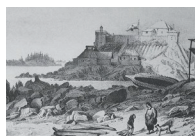
Figure 13.9 Old Sitka, ca. 1827. The most heavily fortified trading establishment on the northwest coast reflects the poor relations its Russian occupants had with Tlingit neighbours.
