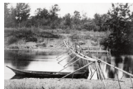
Figure 1.13 Fishing weirs like this one from the Cowichan River (ca. 1866) were built by Aboriginal peoples across Canada long before contact. Wood, a readily available building material in northern North America, was used far more widely than stone, but it leaves less evidence behind. [Long Description]
