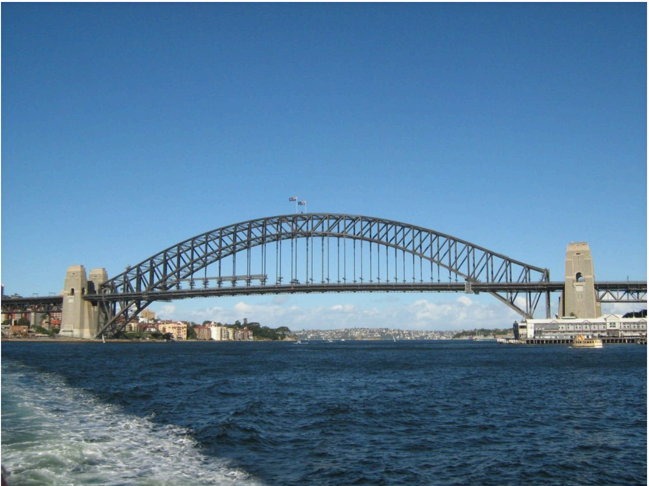
Figure 5.0.1: Blues Point Bridge, Sydney NSW, Australia Photo by Robert Cutts CC-BY-SA 2.0
